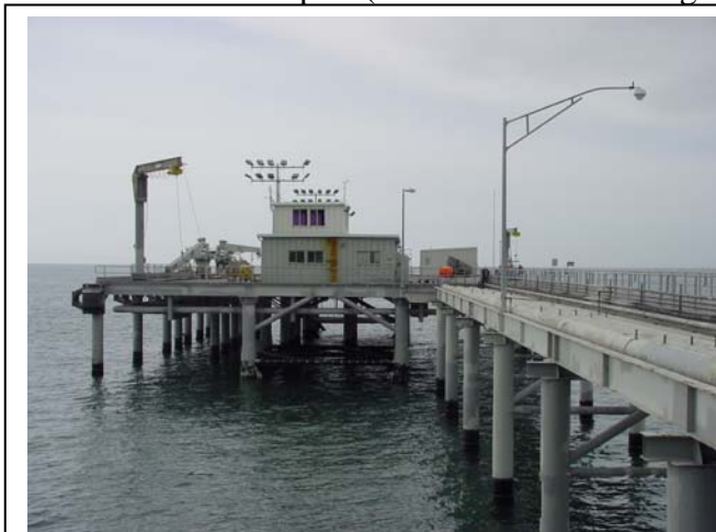
Figure 4. View of main platform, buildings and associated hoists
