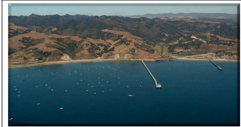
Figure 2. Aerial view of the MERC from the South.
