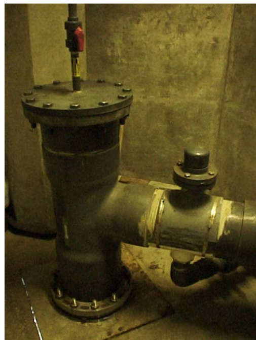
Figure 8. Vacuum intake system at Scripps IO. The
