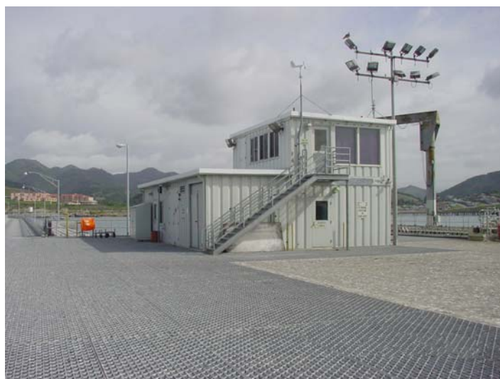
Figure 5. Main building on platform, with dive locker, conference/classroom, machine shop, offices and electrical circuitry.
